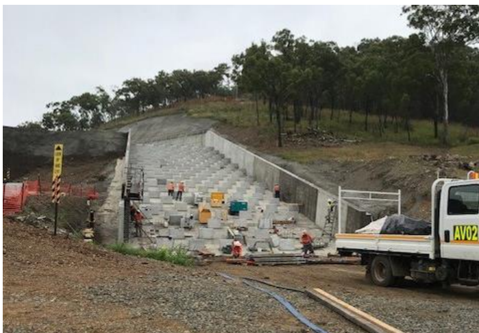
The Offline Water Storage Facility Spillway
