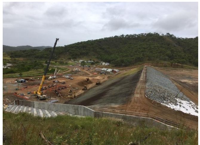
View of the embankment from the northern side
