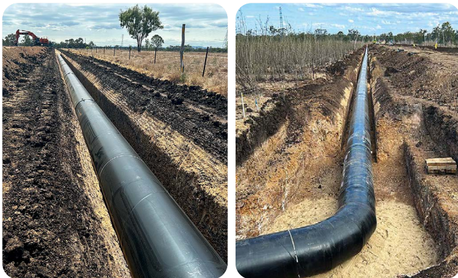
Pipe laid in Alton Downs in the northern pipeline corridor.
