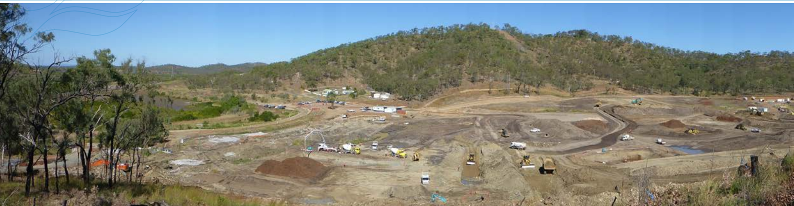
Figure 3: Earthworks in progress for the offline storage and standby pumping system
